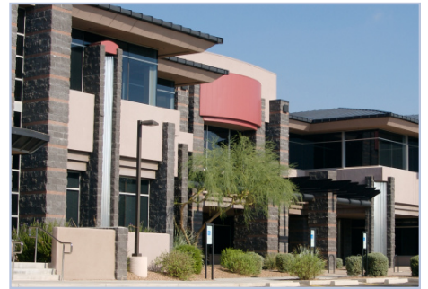
Vegetation too close to windows.
